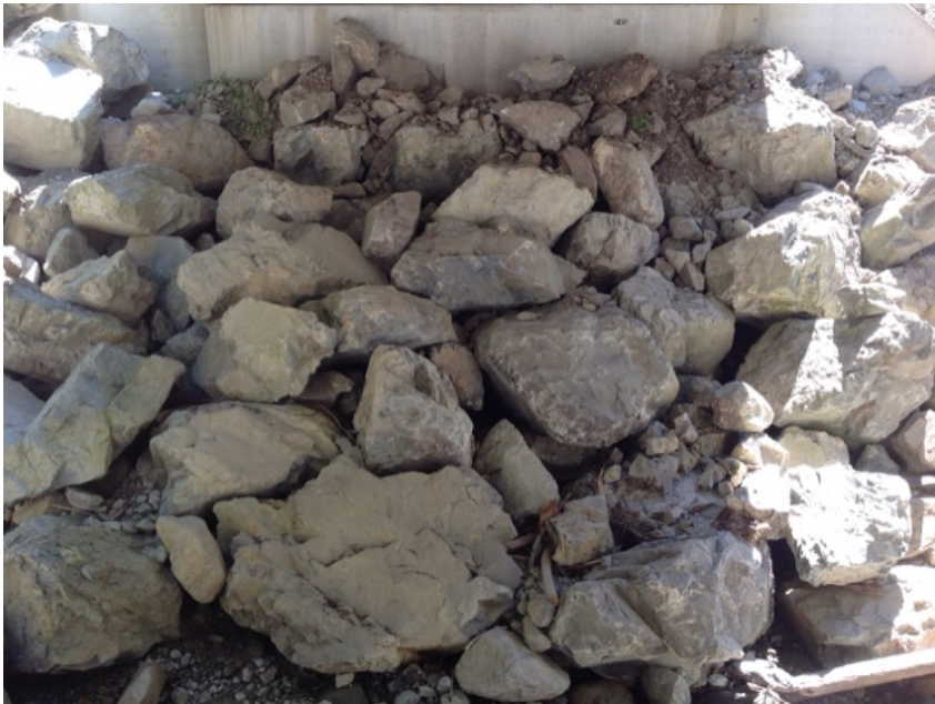
Left Bank Abutment when facing downstream
