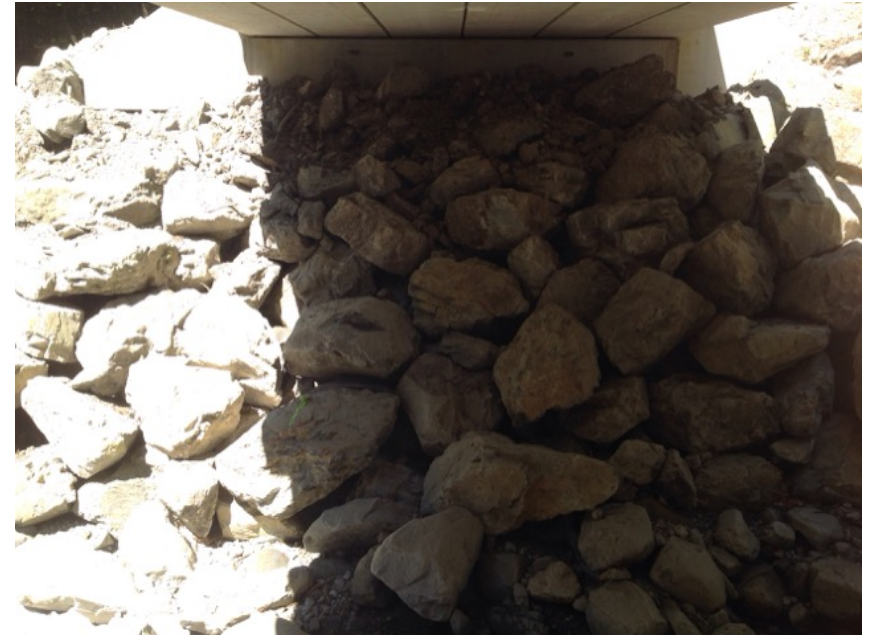
Right Bank Abutment when facing downstream
