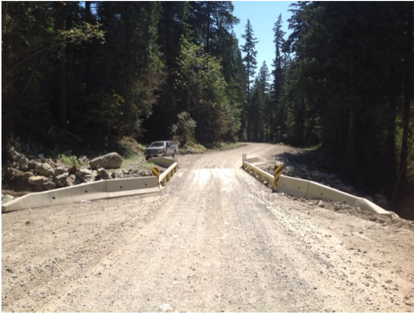
Approach from Right Bank when facing downstream
